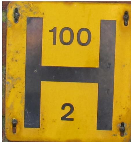
A modern standard hydrant plate, showing the diameter of the water main (in millimetres) in the top section and the distance the hydrant is from the plate (in metres) in the lower section.
